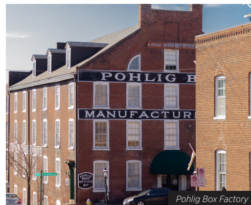
Pohlrigg Box Factory
